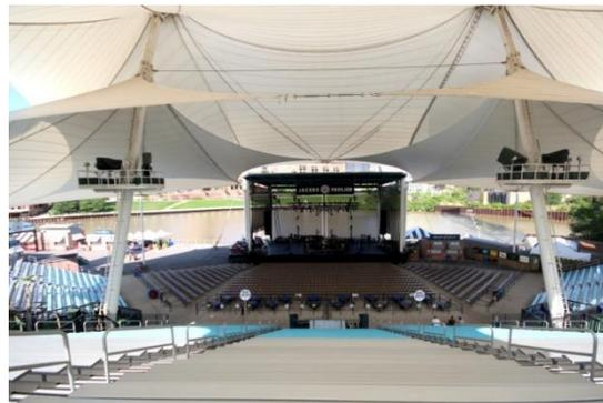
Above is Jacobs Pavilion, in Cleveland. This tensile structure forms a shelter for the amphitheater inside. Tensile membrane structures can easily be grasped by picturing a circus tent. (source: davidgray.com)
